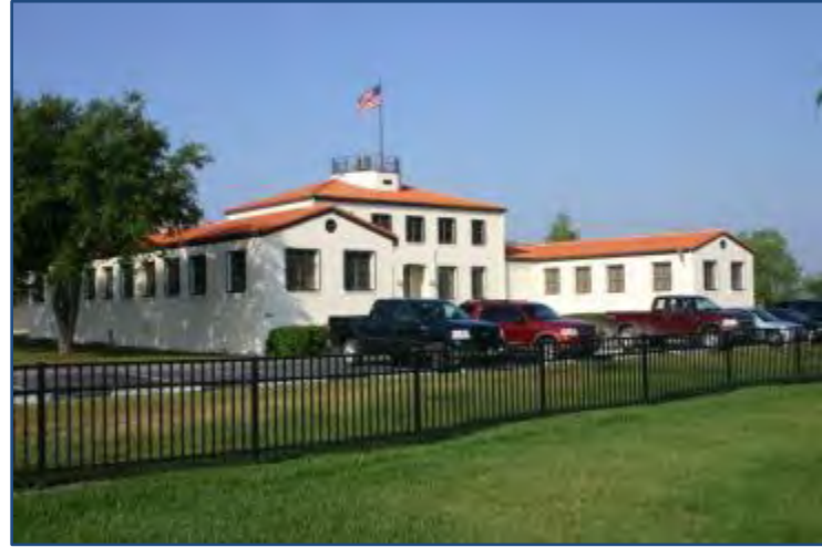
Current administration building, built in sections between 1930s and 1940s and used as laboratories and faculty offices
