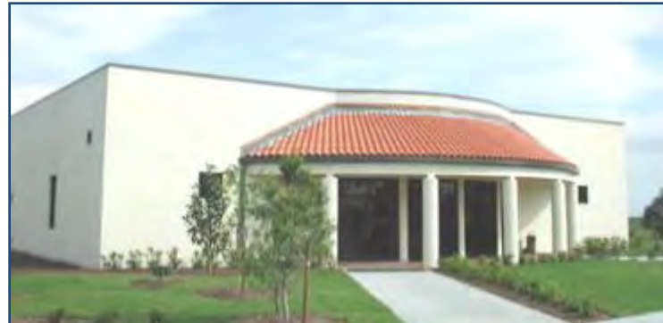
EREC Conference Center for agriculture related meetings, completed in 2001
